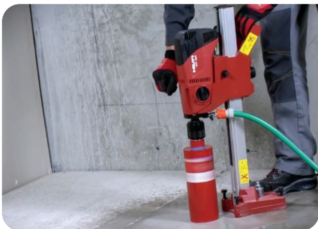
Figure 1. Typical coring setup
