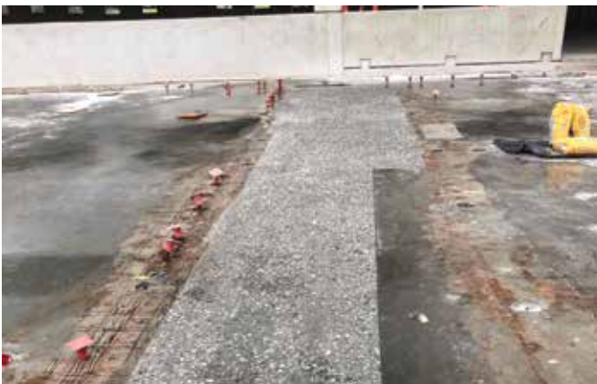
Fig. 6: Most areas required numerous scabbling passes to remove damaged concrete
