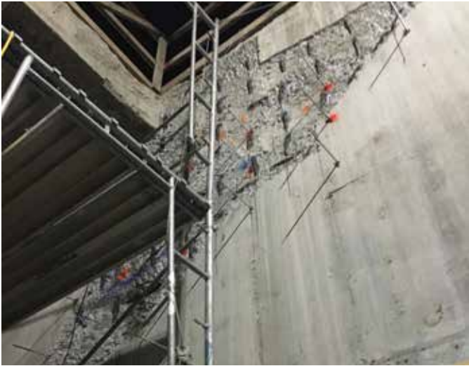
Fig. 7: Vertical patching repair
